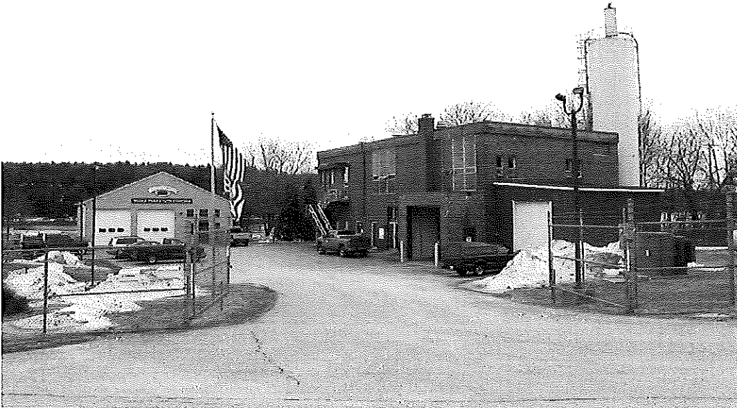
Bath Wastewater Treatment Facility (Portland Press Herald 2018)
