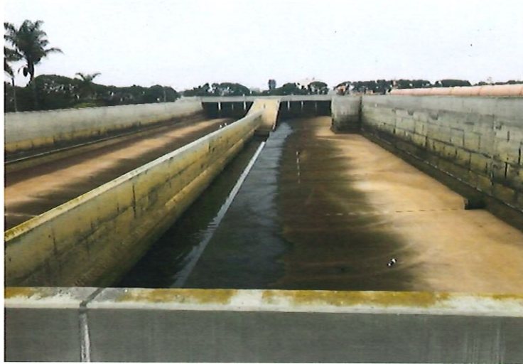
Figure 12: Equalization basins sized to hold 2.5 million gallons.
