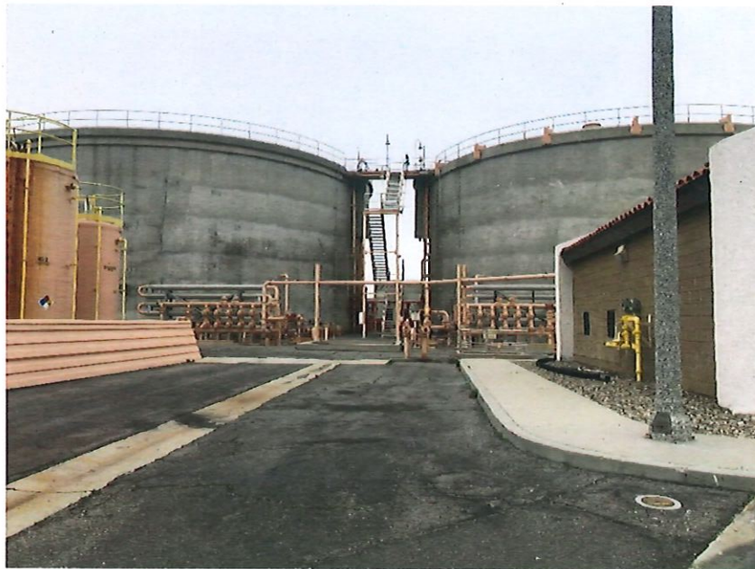
Figure 16: Two of the three anaerobic digesters onsite.
