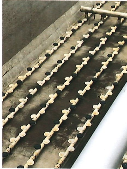
Figure 9: Accumulation of snail shells at base of empty activated sludge tank.
