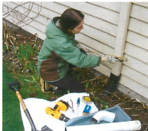
Figure 27. Photo of an Arcata resident disconnecting a storm drain that was connected to the sanitary sewer (CoA 2019e).
