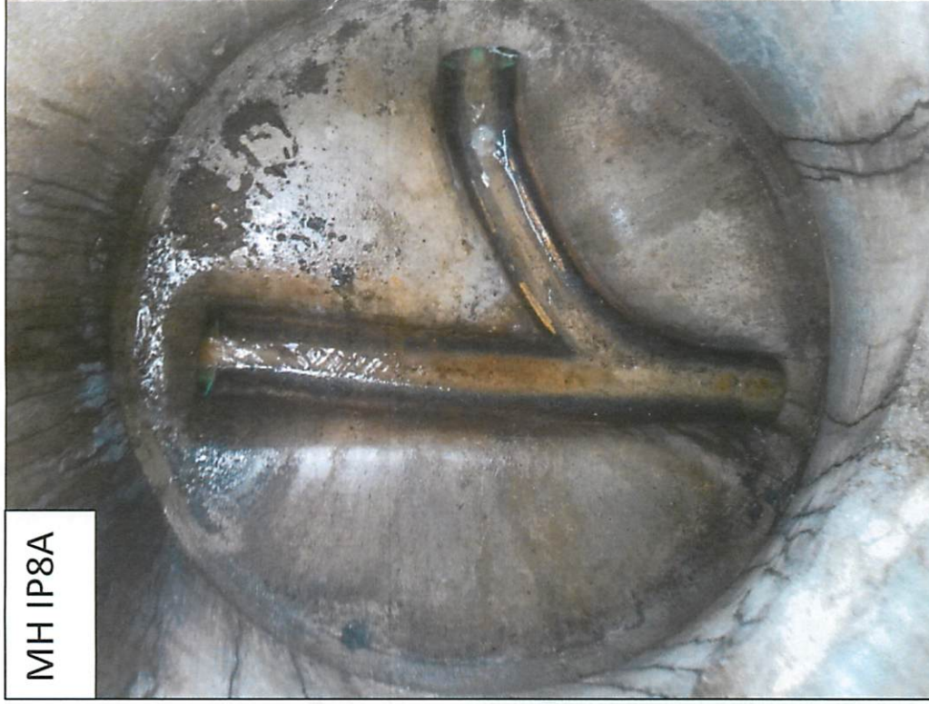
Figure 18. Sanitary sewer manholes connected to the Aldergrove sewer showing signs of infiltration.
