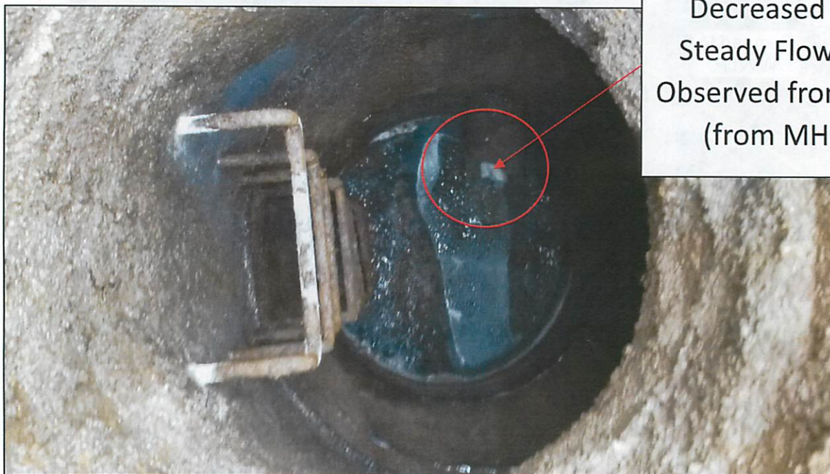
Figure 17. Observed flow response in Manhole IP1 (lift station manhole) when manhole 2 was not plugged (top), and when it was plugged (bottom). Shows that there was still significant flow coming from the pipe down stream of Manhole 2 even though flow into Manhole 2 was plugged.
