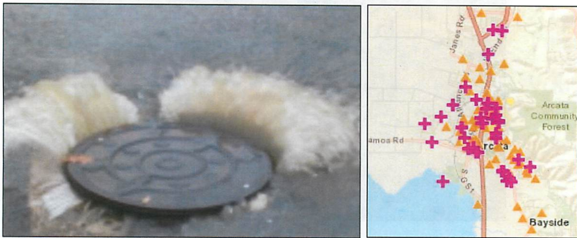
Figure 6. A sanitary sewer over flow in Arcata (left), and the locations of sanitary sewer overflow events in Arcata since 2007. The pink crosses indicate a category 1 overflow, which means the overflowed water reached surface water. The orange triangles indicate SSOs that did not result in surface-water contamination (CoA 2019c) (CA State Water Board 2019).
