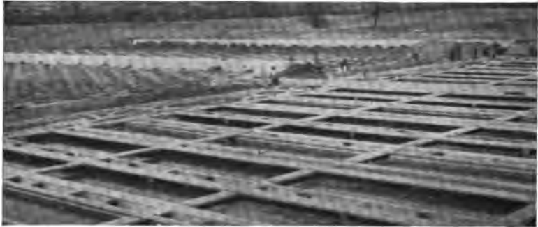
FIG. 41.—IMHOFF TANKS AT SCHENECTADY, N. Y.
