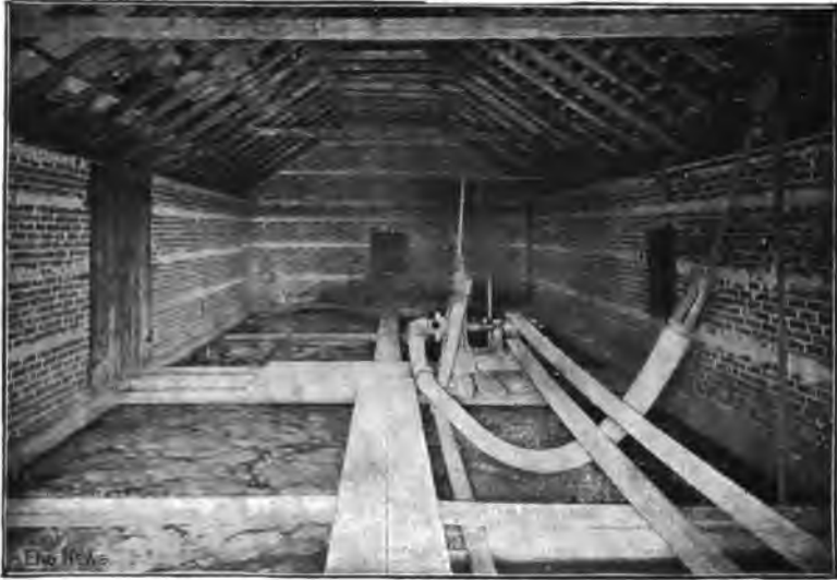
FIG. 38.—INTERIOR OF CHAMPAIGN, ILL., COVERED SEPTIC TANK. (From Engineering News .)
