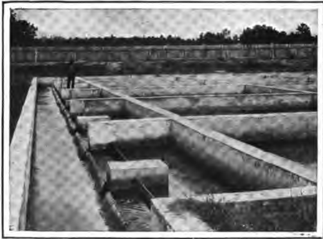
FIG. 39.—DISCHARGE-WEIRS, SEPTIC TANKS, BIRMINGHAM, ALA. (From Municipal Journal and Engineer .)
